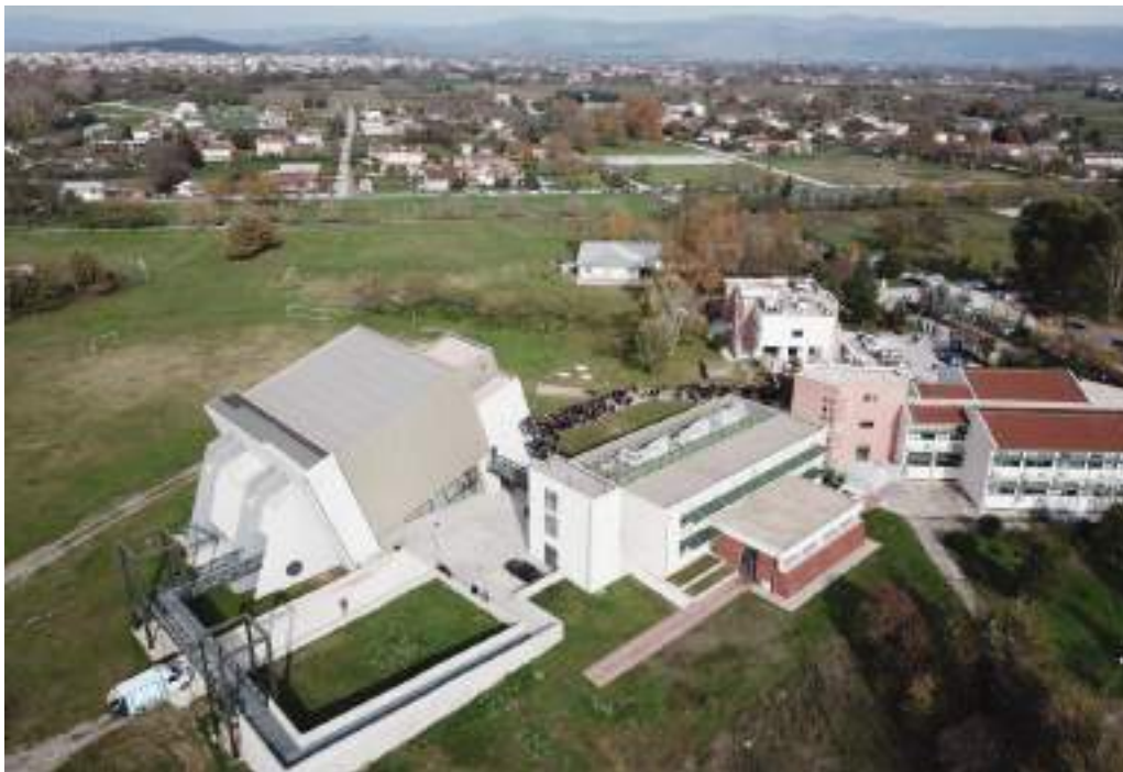
Photo of the facilities and premises of DPESS.
