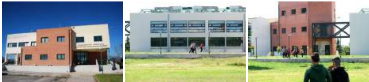
Part of the DPESS facilities.
