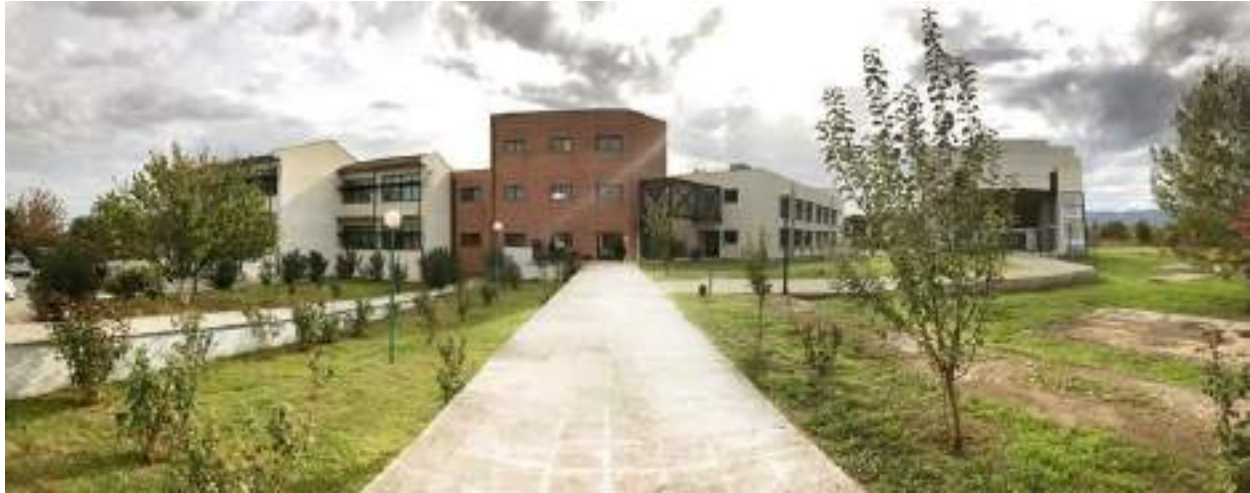
Part of the DPESS facilities.
